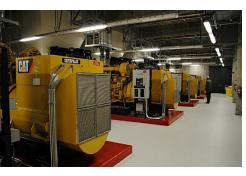
Total Cost: \$27 Million Generator Plant: 25,000 SF Hospital: 1.5M SF Location: Anchorage, Alaska Owner: PAMC Project Completed: 2015 AMC was the Prime Consultant for PAMC's new 8 MW diesel power plant and reconfiguration of the power distribution system that serves the Essential Electrical System (EES) for the existing main hospital facility and the new "Generations" addition.
